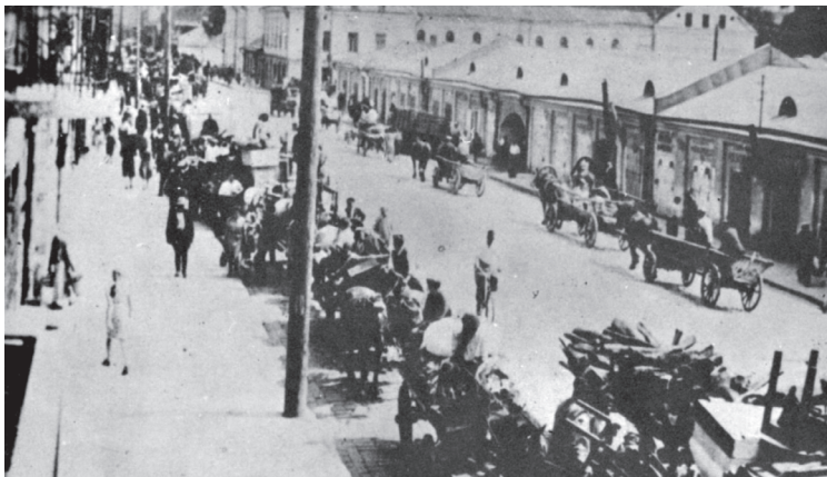
The creation of the Kaunas Ghetto: Jews forced to leave the city for the suburb of Vilijampolė (Slobodka) in August 1941.
